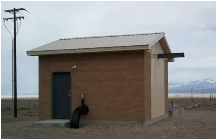
Photo #2 Cutline: Except for this small power house and adjacent power line, passers-by would not even know the RO Ranch hydro power project existed.
