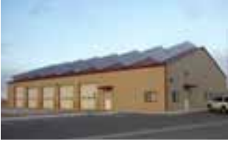
Solar array in Ely.
