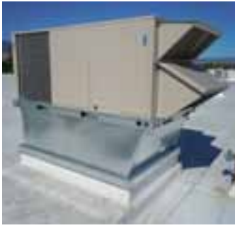
New HVAC system at Truckee Meadows Community College.
