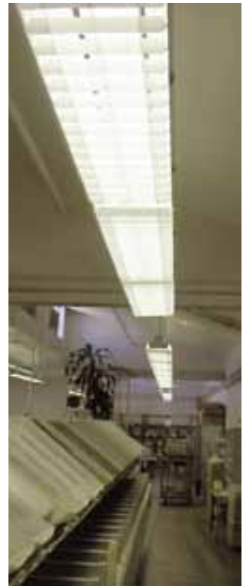
New, energy efficient lighting in the state printing building has helped reduce electrical usage.
