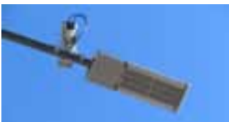
LED street light in Carson City.
