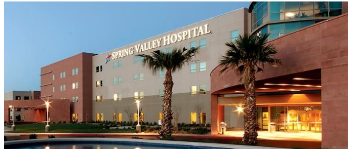
Valley Health Systems in Clark County earned one LEED Gold certificate and received a GOE incentive for the energy efficient upgrades made to their 359,103 square feet medical center.
