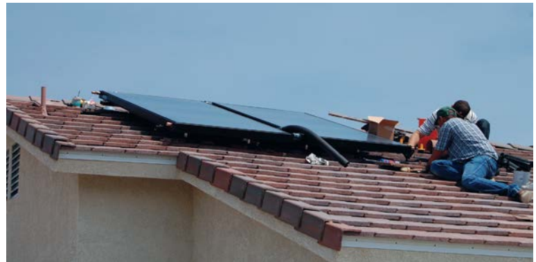
Workers mount two solar panels to the roof of a home in Pahrump while installing a solar water heating system from Valley Electric Association.
