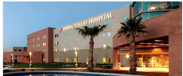
Valley Health Systems in Clark County earned a LEED Gold certificate and received a GOE incentive for the energy efficient upgrades made to their 359,103 square foot medical center.
