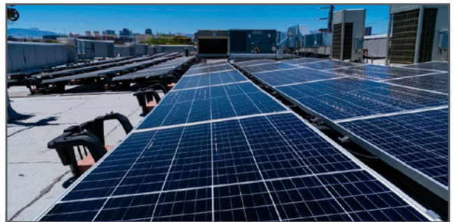
HELP of Southern Nevada's Shannon West Homeless Youth Center received LISEP funding in 2019 for a solar installation on the 37,000 square foot housing facility with capacity to house 150 youth. Despite a more than 30 percent increase in youth housed at the center, their electric bills have been reduced by nearly $18,000 since the solar panels were installed in 2020. These operational savings allowed HELP to open their third floor, providing some rooms as a COVID-19 isolation area. Photo courtesy of NV Energy.
